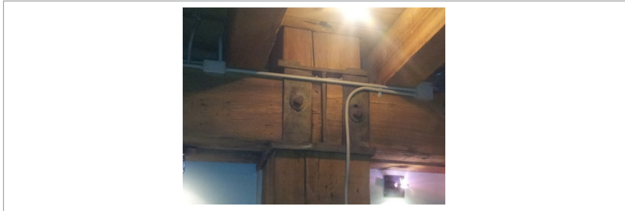
Figure 5-25: Photograph of a 1908 column connection designed to be “fail safe” under gravity loads. Failure would result in wood crushing but not structural collapse
