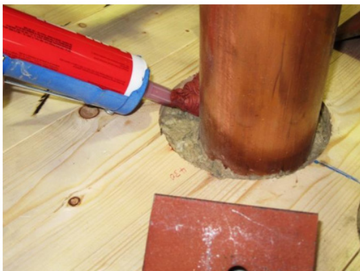
Figure 5-48: Photograph of an upper 12.7 mm annular space filled with mineral wool and caulking, and steel sleeve filled with intumescent caulking
