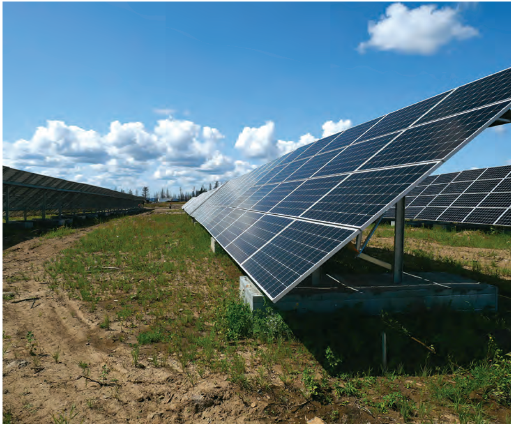
Because of its northern location, the modules of the Tsilhqot'in Solar Farm had to be angled to about 45 degrees. PHOTO: EcoSMART FOUNDATION INC.
