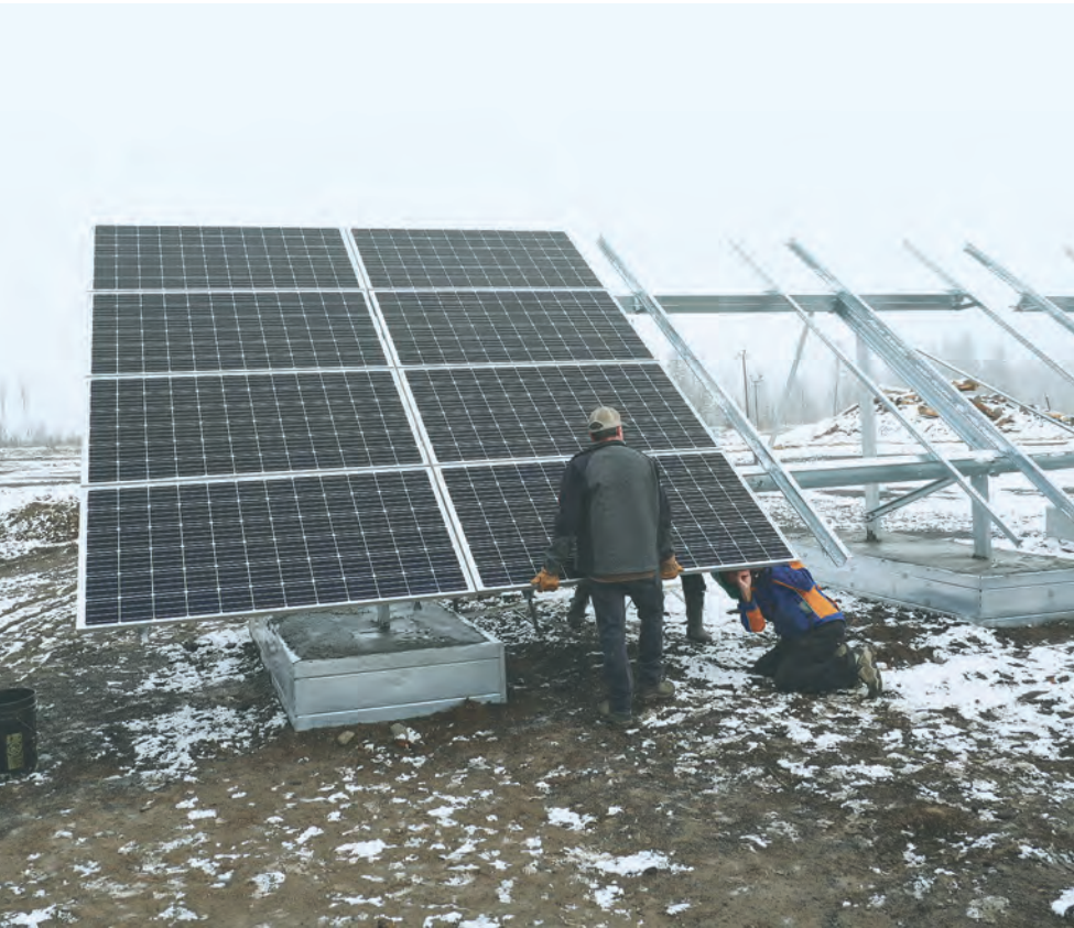
Workers install solar photovoltaic modules on custom racks. PHOTO: EcoSMART FOUNDATION INC.
