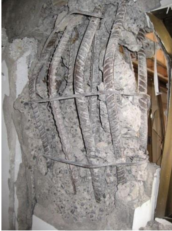
Column rebar buckling damage – Probable replacement
