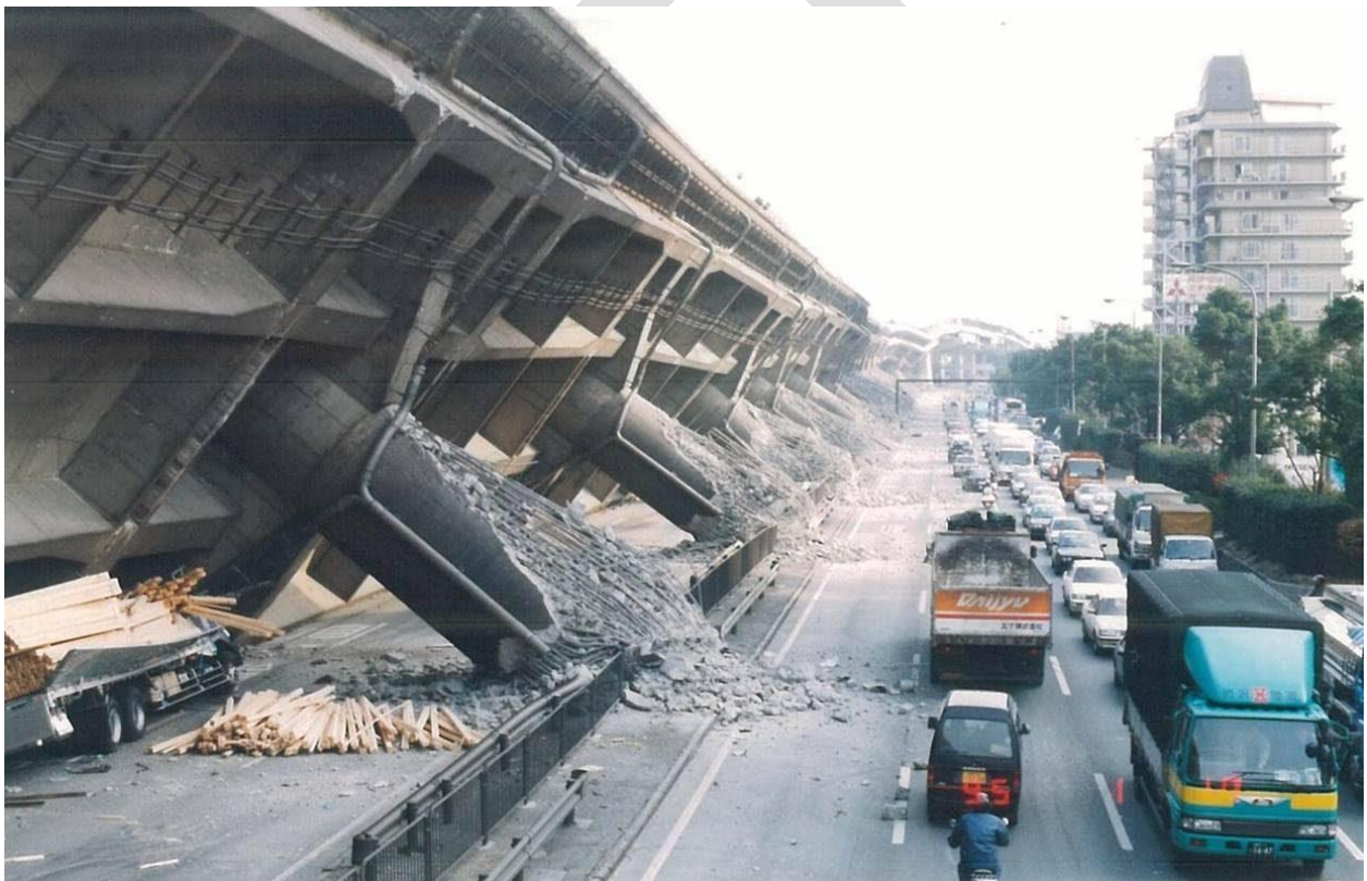
Hanshin expressway collapse due to premature longitudinal rebar termination and lack of confinement reinforcement
