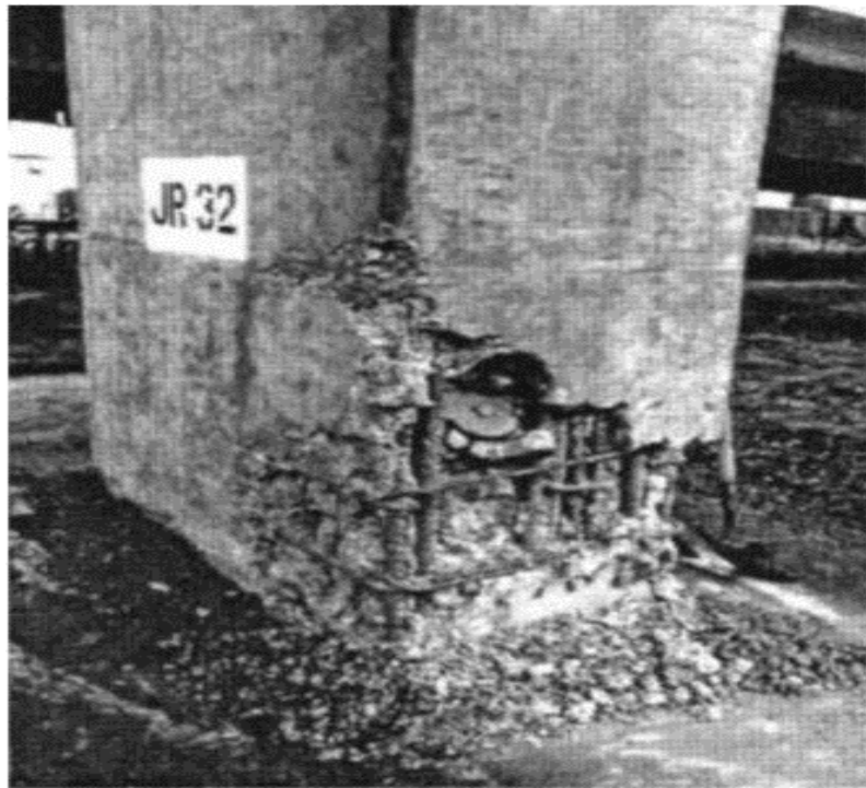
Extensive damage due to plastic hinge lap-splice failure
