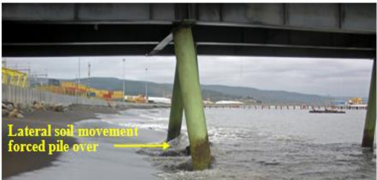
Kinematic load on pile (FHWA Report, 2011) – Probable replacement
