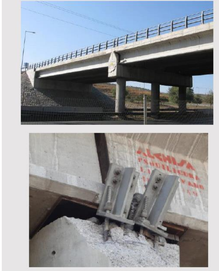
Shear key failure – Repairable Damage
