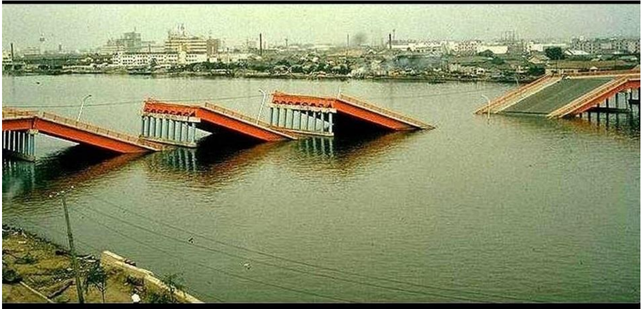
Lateral spreading induced simple span collapse
