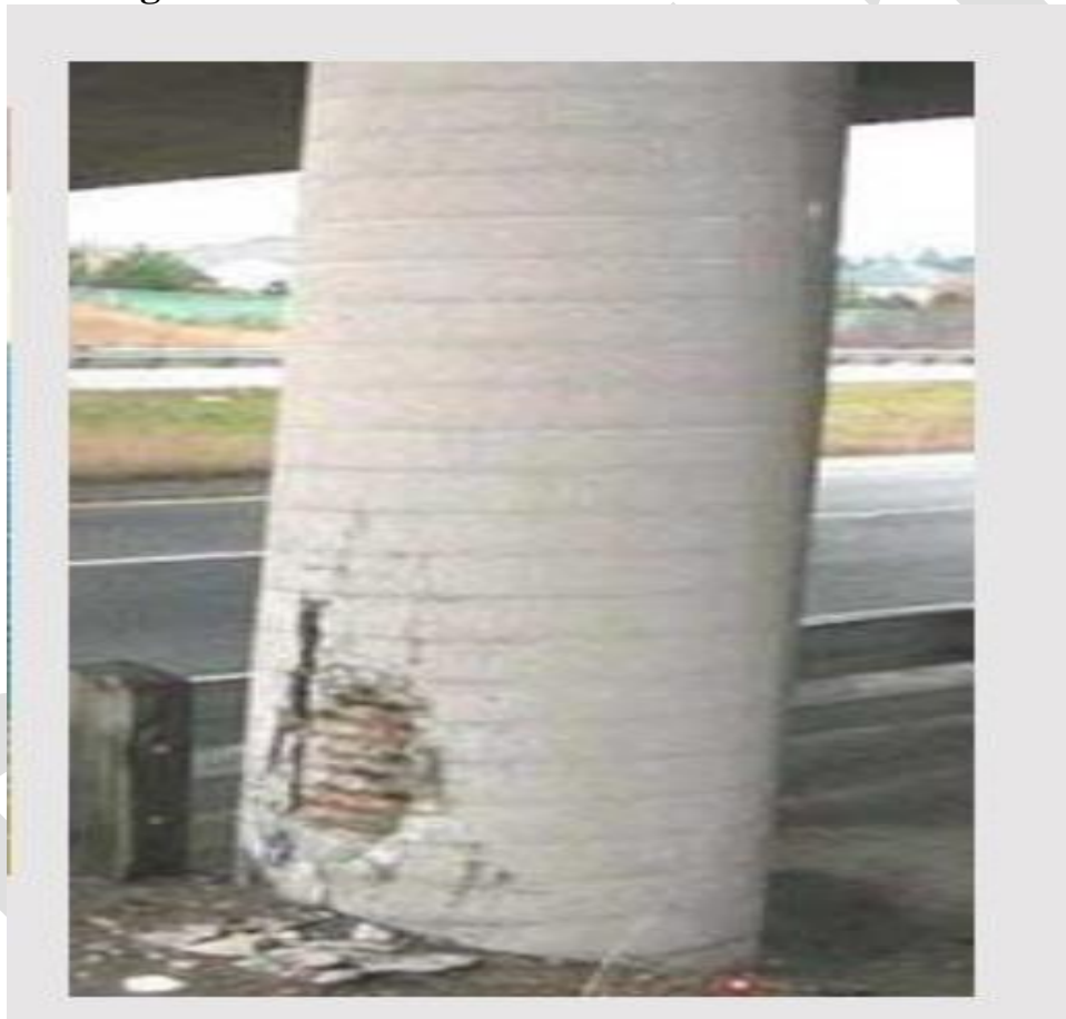
Minimal column damage – onset of spalling
