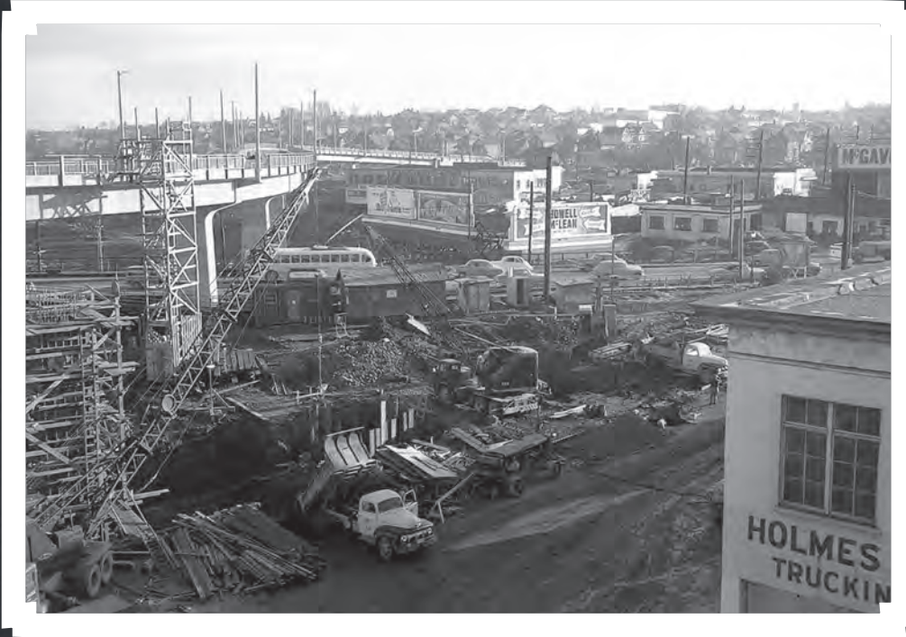
The 1953 version of the Granville Street Bridge (an eight-lane structure) was actually the third Granville Street Bridge. The first (a trestle design) was built in 1889, and the second in 1909. CITY OF VANCOUVER ARCHIVES, CVA 228-332. PHOTO: LEW PARRY FILM PRODUCTIONS.
