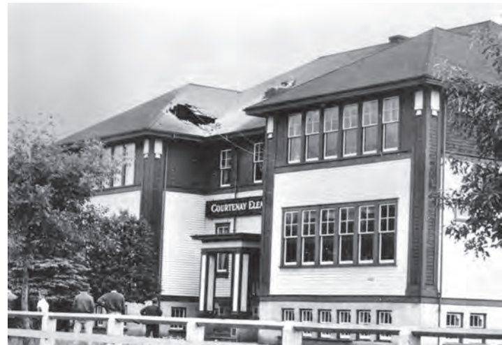
Damage at Courtenay Elementary after an earthquake in 1946. The hole in the roof in the photo on the left was caused by a chimney collapsing. GEOLOGICAL SURVEY OF CANADA, NATURAL RESOURCES CANADA ( WWW.EARTHQUAKESCANADA.NRCAN.GC.CA/HISTORIC-HISTORIQUE/EVENTS/19460623-PHOTO-EN.PHP )
