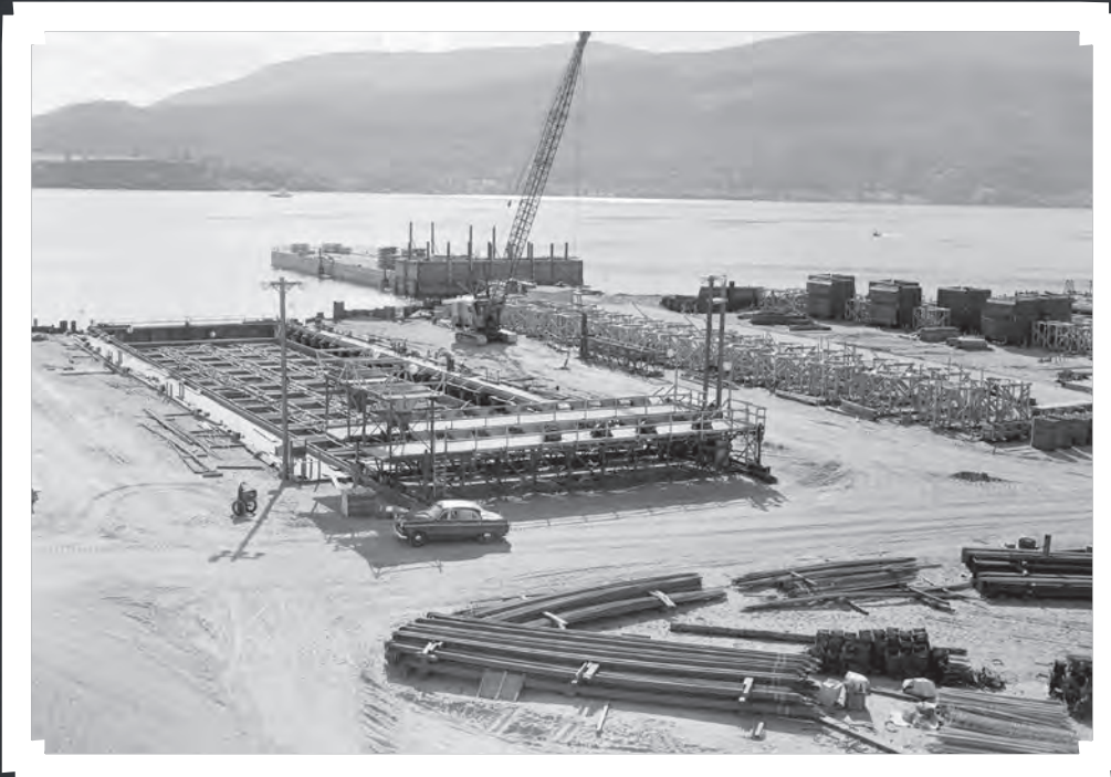
The Kelowna Floating Bridge (formally known as the Okanagan Lake Bridge) was a three-lane, 650-metre pontoon bridge with a vertical lift, that crossed Okanagan Lake. Operational in 1958, the bridge was the first of its kind in Canada. It was replaced by William R. Bennett Bridge—also a pontoon bridge—in 2008, and then dismantled. VANCOUVER PUBLIC LIBRARY SPECIAL COLLECTIONS, 41380. PHOTO: WILLIAM CUNNINGHAM, PROVINCE NEWSPAPER
