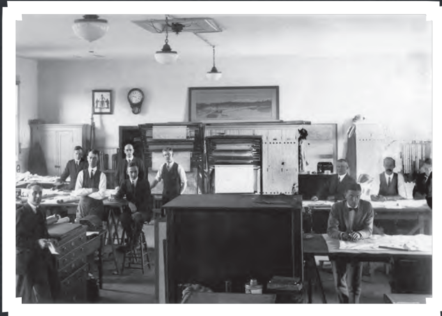
Engineering staff (surveyors, drafters, and sewer systems engineers) in the south wing of the City of Vancouver's Main Street office. City staff would move to an East Hastings building five years later, and then to its current location on 12 th Avenue in 1936. CITY OF VANCOUVER ARCHIVES, CVA 216-6
