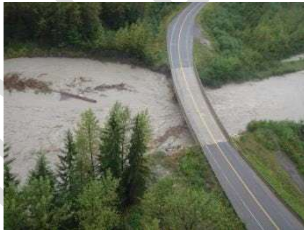
Figure 1. Looking down at Bitter Creek Bridge on Highway 37A just prior to the washout of its west abutment in September 2011- flow is left to right (September, 2011).
